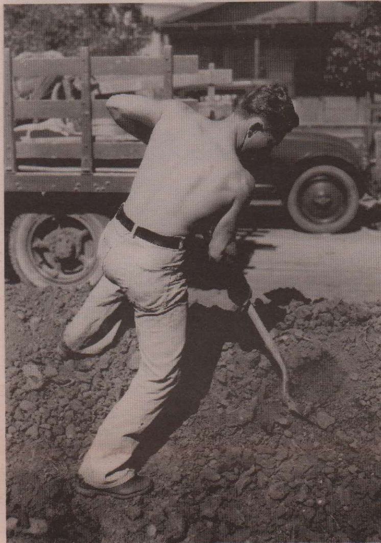
Worker on a New Deal Public Works Administration project in Los Angeles
